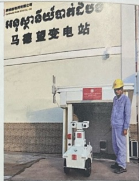
An intelligent patrol robot at the Battambang Substation invested and built by the China Datang Corporation can perform 24/7 intelligent inspection and monitoring of the substation. (DONGHUA DAILY)
